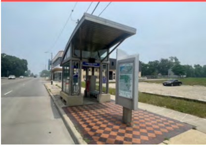
HealthLine BRT station in Circle East District.
